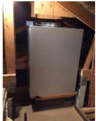
Accordingly a new fan was purchased to replace the one in the roof. This fan presented a challenge: how were we going to get it into the roof? It weighs 63 kilos (140pounds). A block and tackle was hired being capable of lifting one ton. The loft ladder was temporarily removed and a beam was screwed between two rafters directly above the loft hatch. The fan was duly hoisted into the loft (top left) and manoeuvred into position (bottom left).
